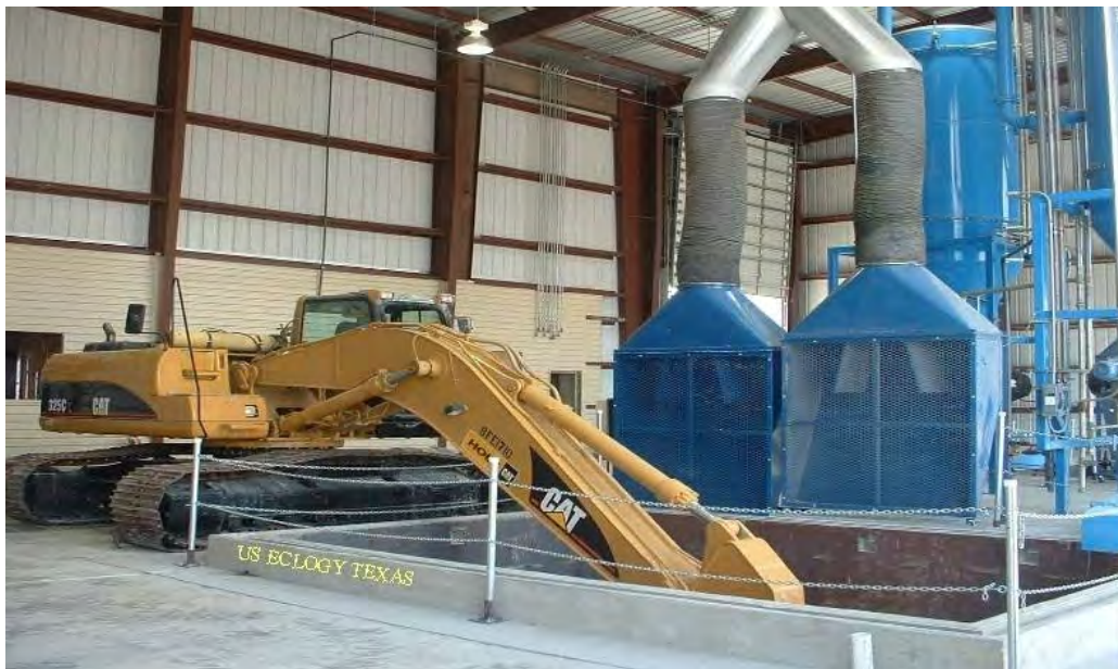
Figure 5 – Mixing wastes in treatment tank (Courtesy of USET)
